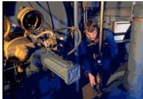
Pressure Leak Check Using Sniff Probe
